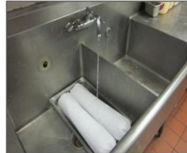
Use of Water to Defrost Food Savings: $450/yr
