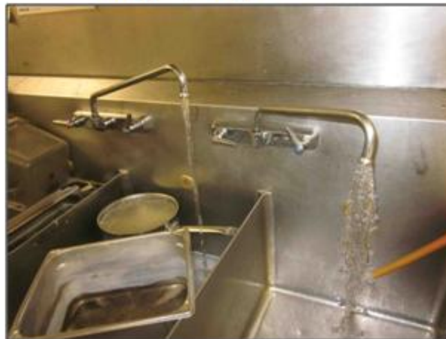
Faucet Aerators Savings: $2,400/yr
