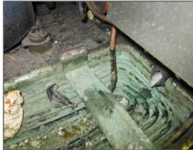
Dirty Refrigeration Coils Savings: $125/yr
